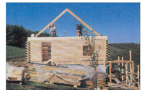
Installing Roof Rafters
