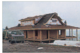
Nailing Roof Shingles
