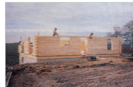
Installing Header Logs
