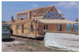
Installing Dormers & Porch
