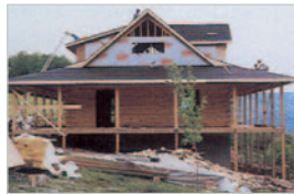
Applying Roof Felt
